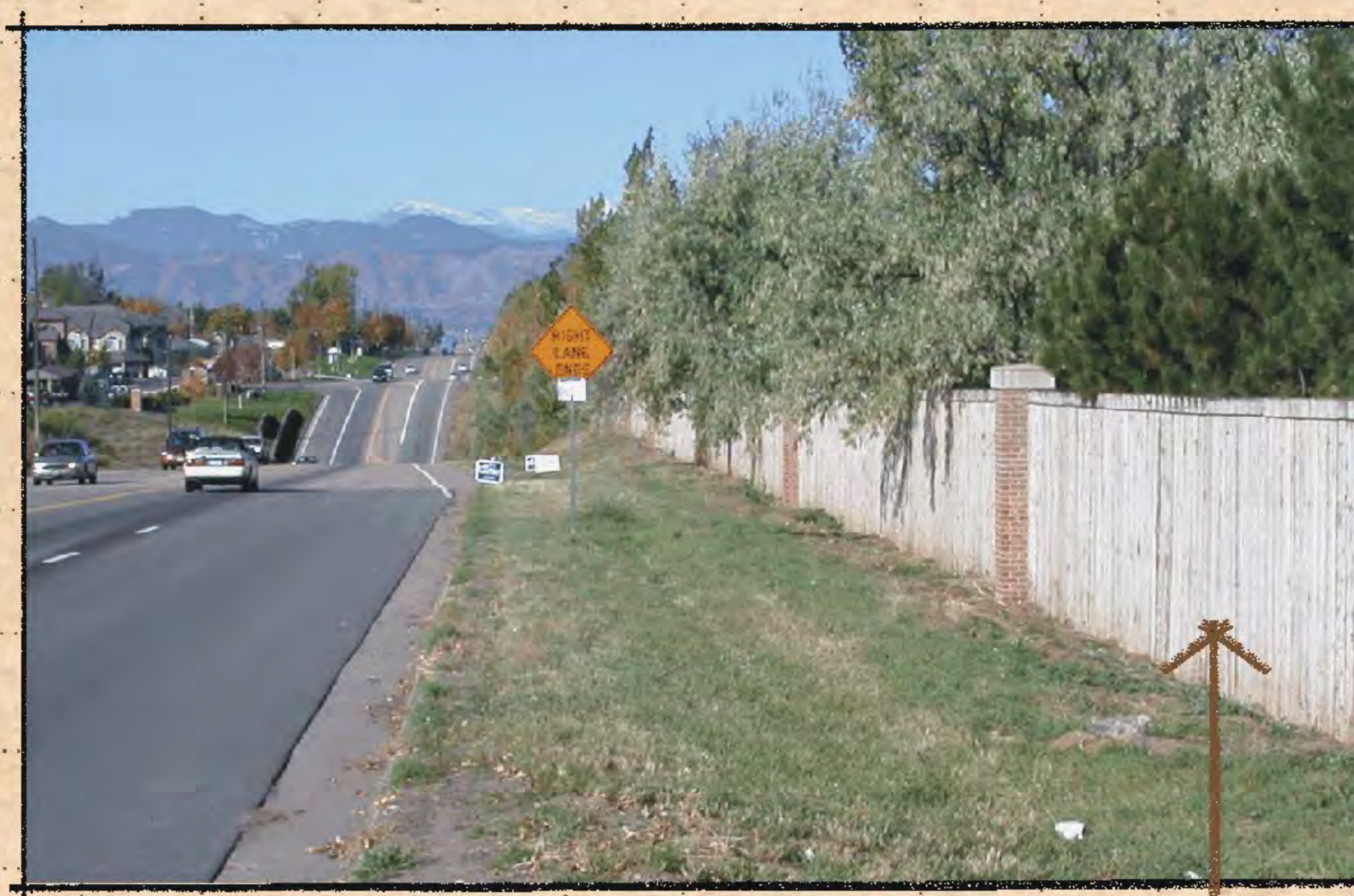
Photo of solid wood fence with masonry columns. Although the masonry columns give it some refinement it has most of the disadvantages of a plain wood fence with minimal sound attenuation and a short life span.
