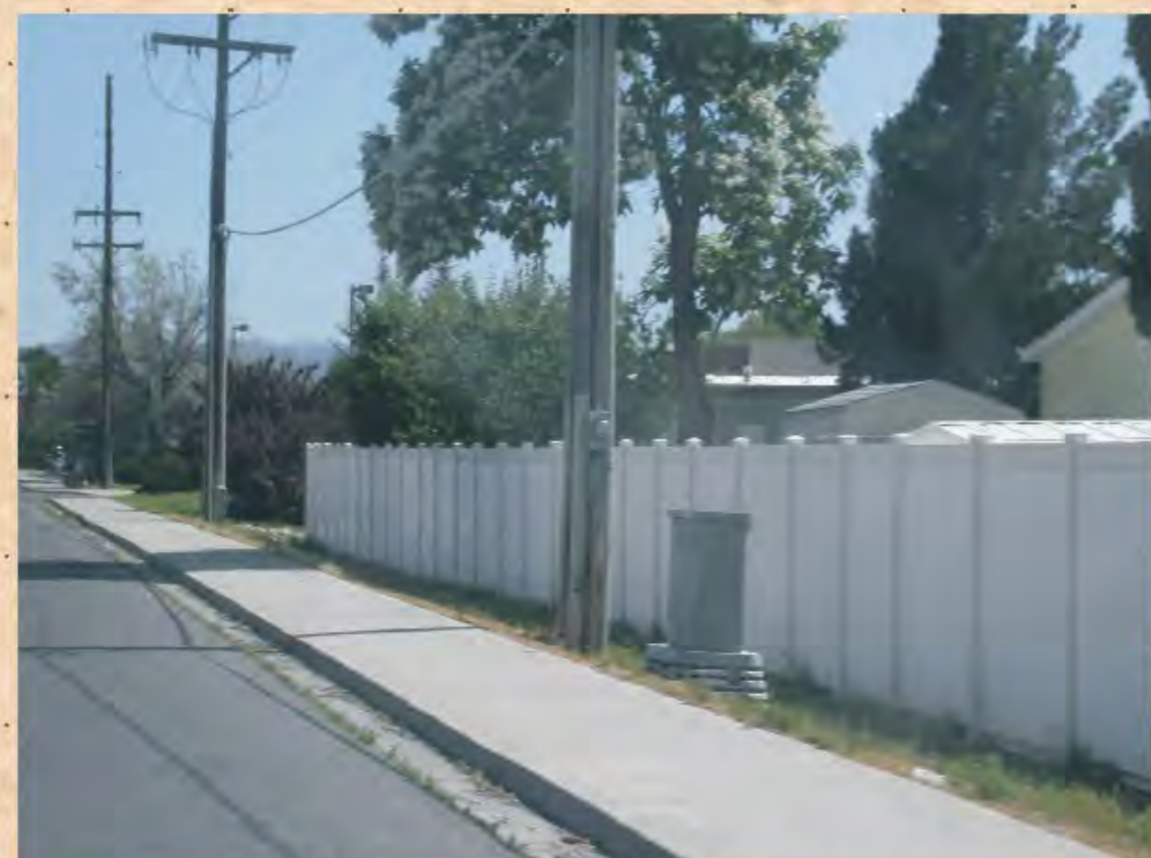
Another solid vinyl fence about 4 ft in height. This one is in shadow. In the bright sun the shiny reflective surface can be rather harsh. Note landscape space in front of fence. Large shrubs should be planted here to soften the view of the fence texture and enhance roadway.
