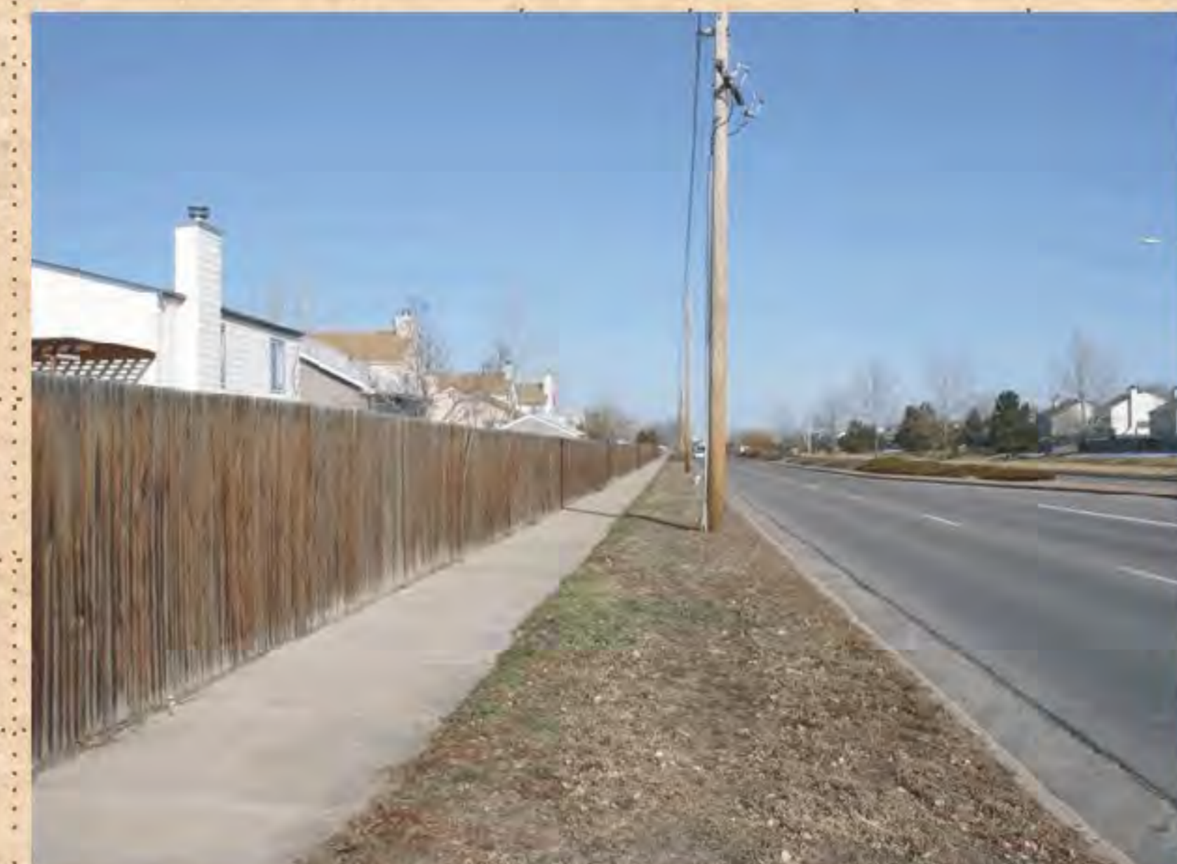
6 ft tall solid cedar fences are popular inexpensive options that have been overused in the past 30 years. Unfortunately these fences only last about 15-20 years. Along this arterial roadway the deteriorating fences become a neighborhood landscape blight issue. These are all private fences, some may get replaced others may not. What is most unfortunate is that there is no landscape space directly in front of the fence to soften the view of the tattered fences.
