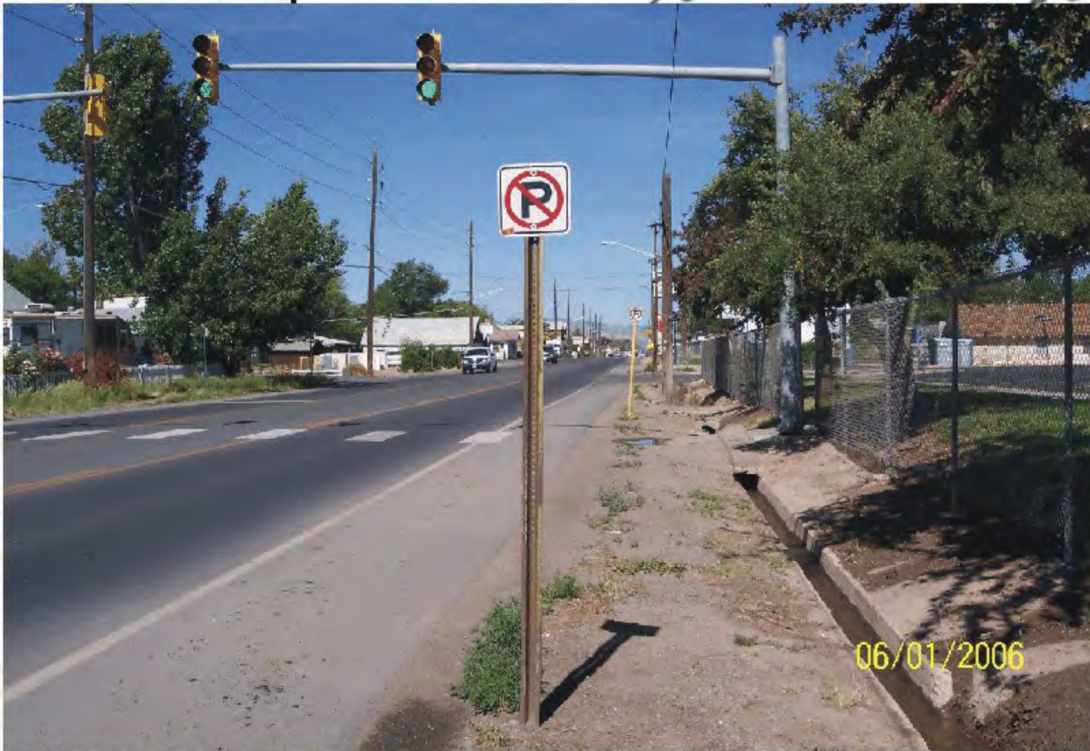
LEFT: Looking west along north side of F Road note wide paved shoulder and irrigation ditch
