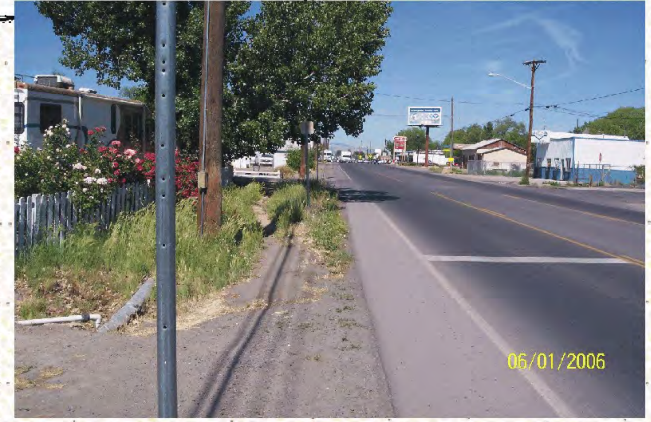
Looking west, south side of F Road near the Clifton Elementary School.
