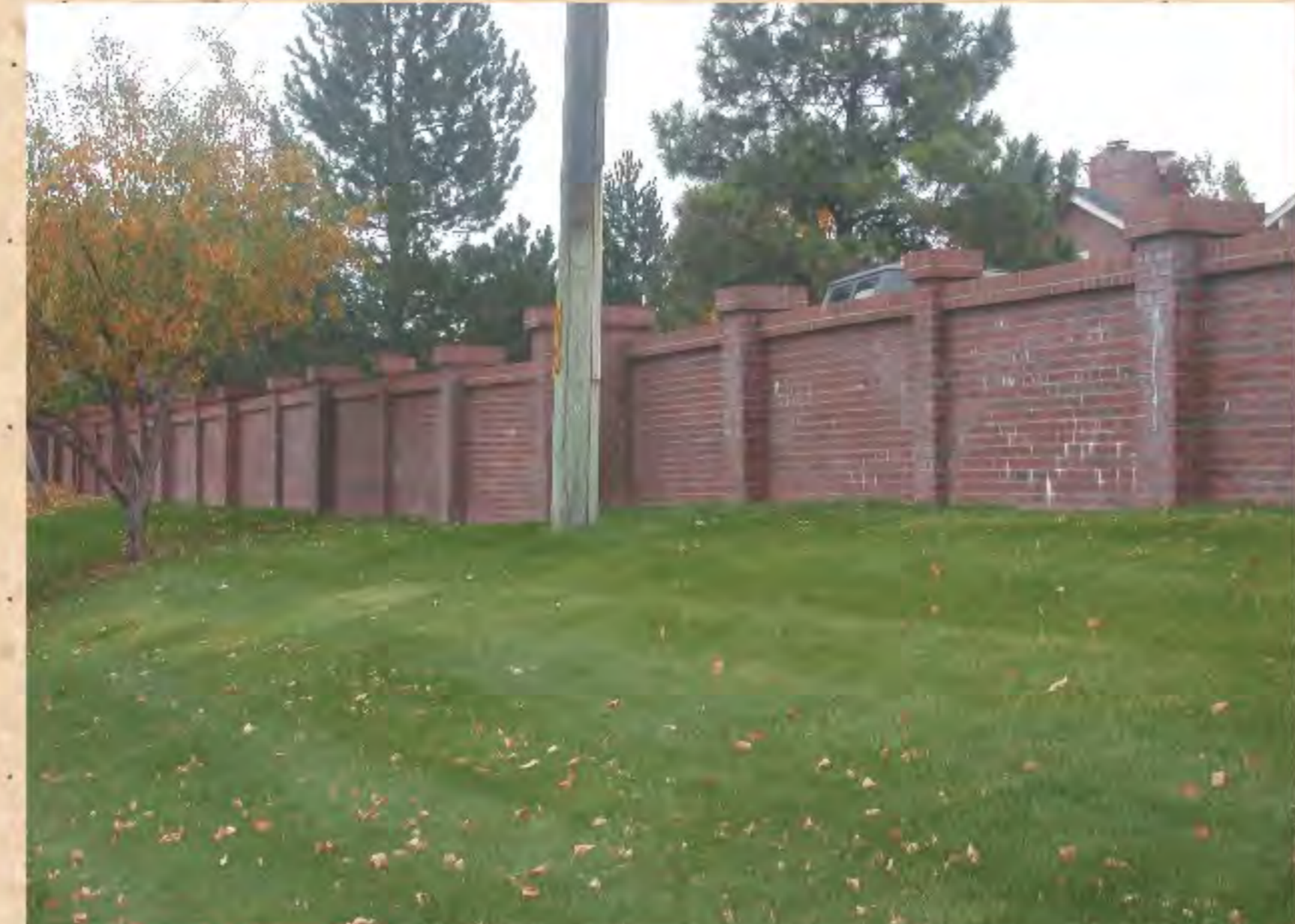
This is a brick masonry wall about 4 1/2 ft tall at the top of a berm separating a parking lot from an arterial roadway. If a fence or wall is desirable this is a high quality attractive solution. Higher masonry walls, whether brick or block should have adequate landscape space in front of the wall for shrub planting.
